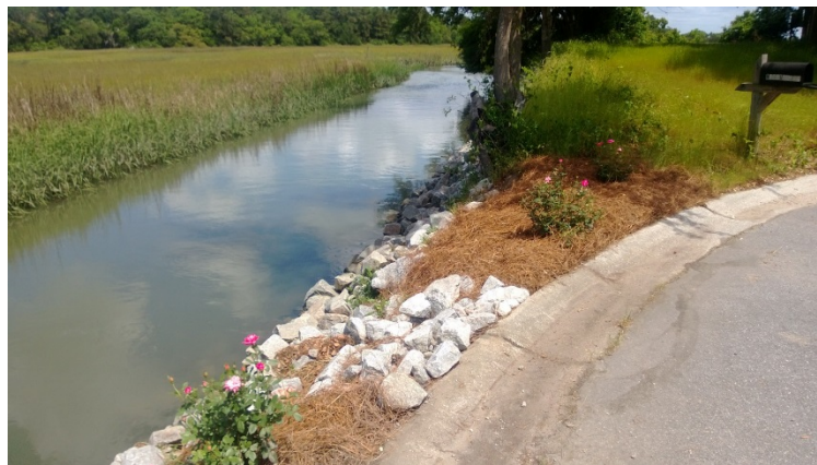
Sweetgrass Creek Erosion Control Project
