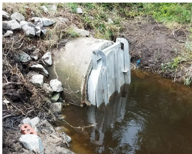
Check Valve Installation
