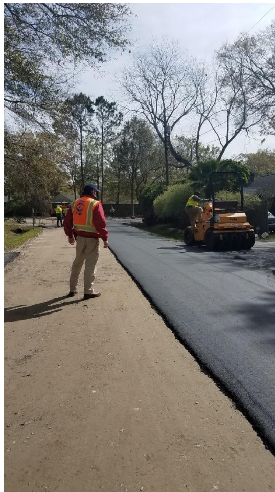
Rembert Rd Paving Project
