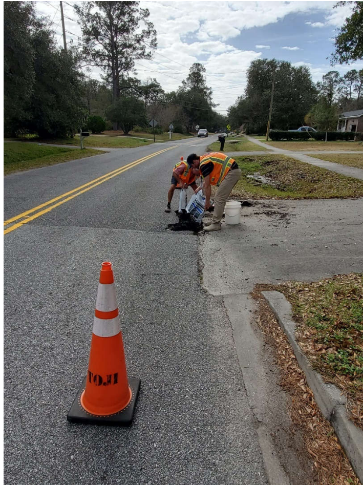
Repairing Pothole on Mikell Dr.
