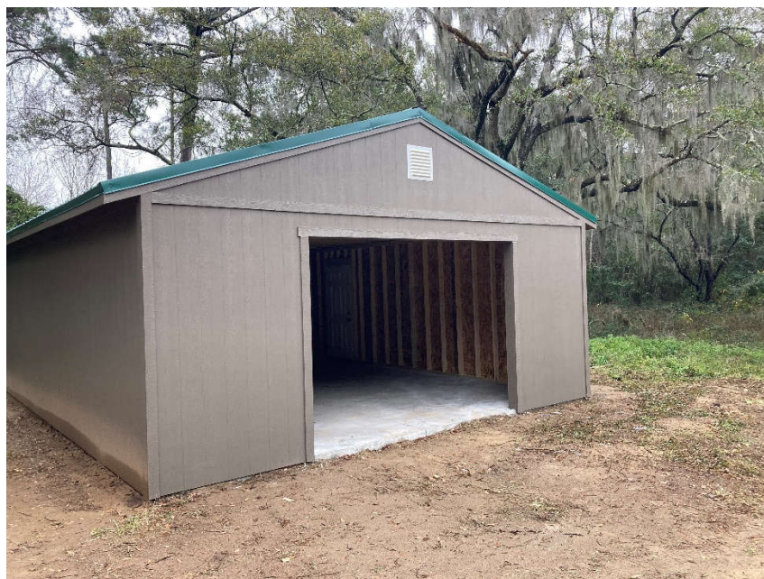
Maintenance Shed at Pinckney Park
