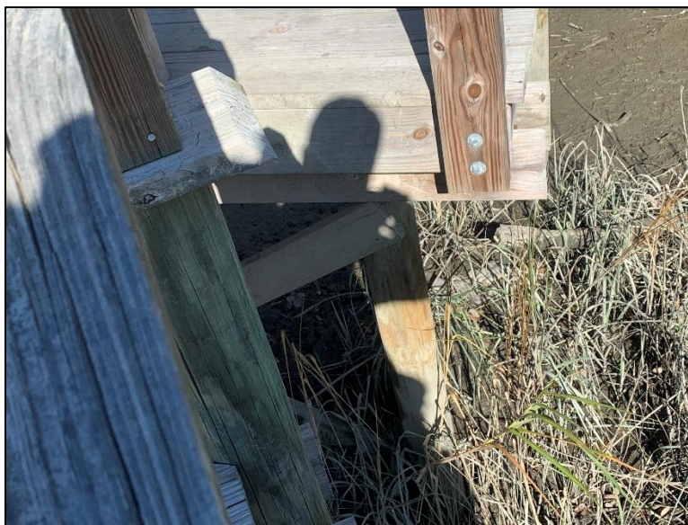
Figure 2.12. Cross-Bracing in One Direction at Bents
