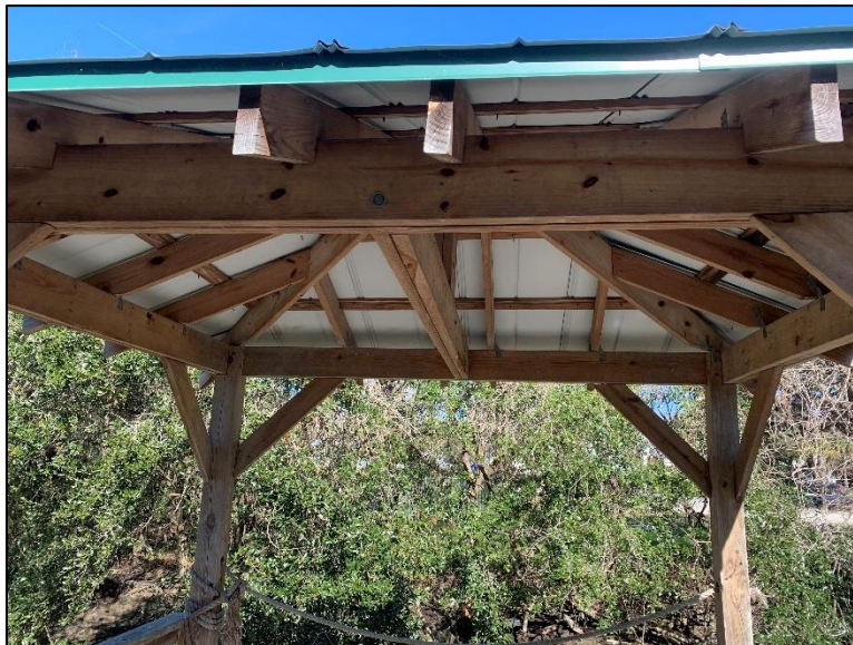
Figure 2.9. Post and Beam Supporting Rafters at Ridge
