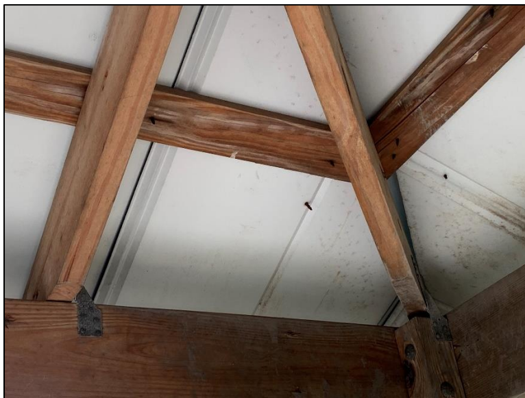
Figure 2.6. Rafters with Hurricane Ties at Ends along the Roof Eave
