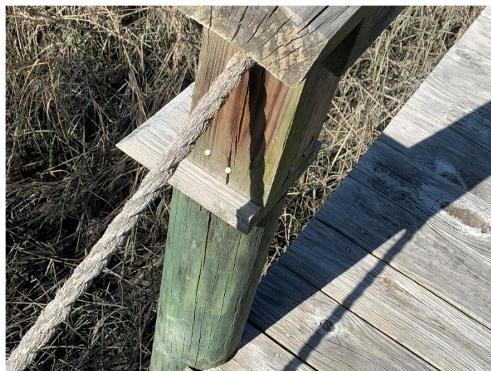
Figure 3.2. Toe-Nailed Railing Post Connections
