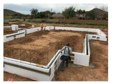
(example of a stem-wall foundation; similar construction to an "elevated slab" where it appears to look like a crawl space is being constructed but after the form is made it is backfilled with dirt and the new slab is constructed on top)
