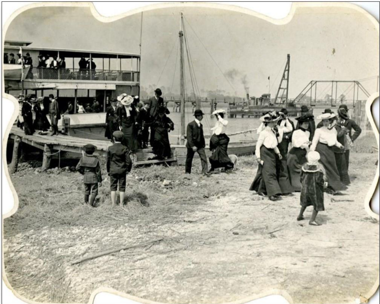
Figure 12.6. 1903 Picture of a ferry at the McLeod landing for the annual Agricultural Society picnic. Note Wappoo Bridge in the background which opened in 1899. The wooden bridge had a single lane metal draw visible along with structural items enabling it to rise for boat traffic. Picture courtesy of the Charleston Museum.
