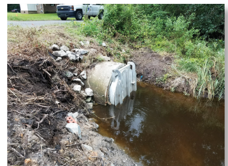
New valve installed by the Town on Sea Aire Dr helps prevent tidal waters coming into the neighborhood
