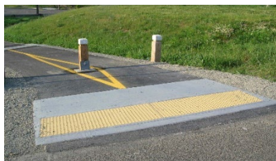
Image 5: Curb ramp with bollards
