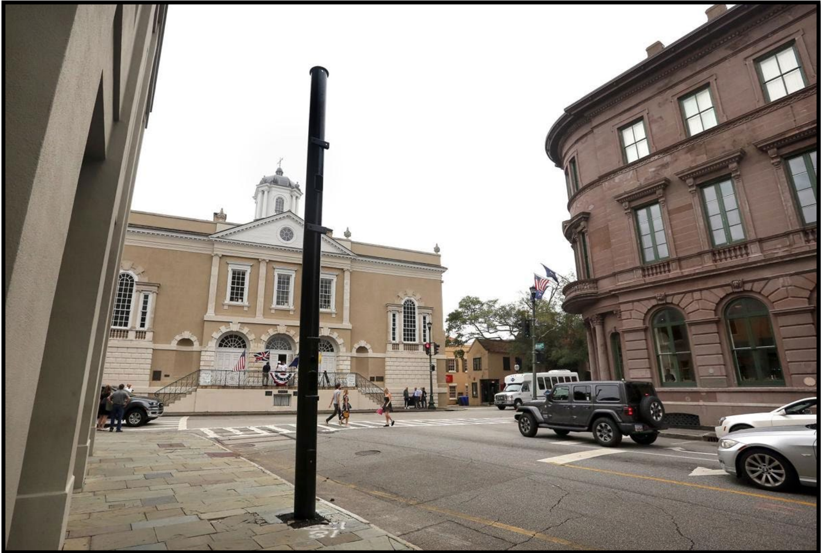
Small cell facility (slim line pole) in Charleston, SC
