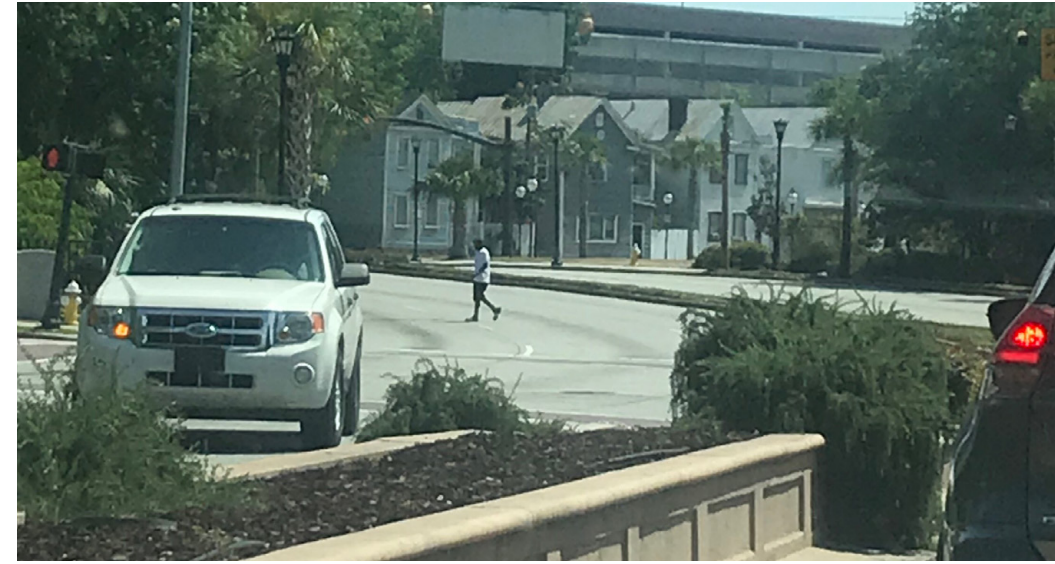
The Septima P. Clark Parkway is an urban highway constructed in the 1960's that divided a predominantly Black neighborhood and displaced many residents in the process. Image courtesy of Becca Hopkins.
