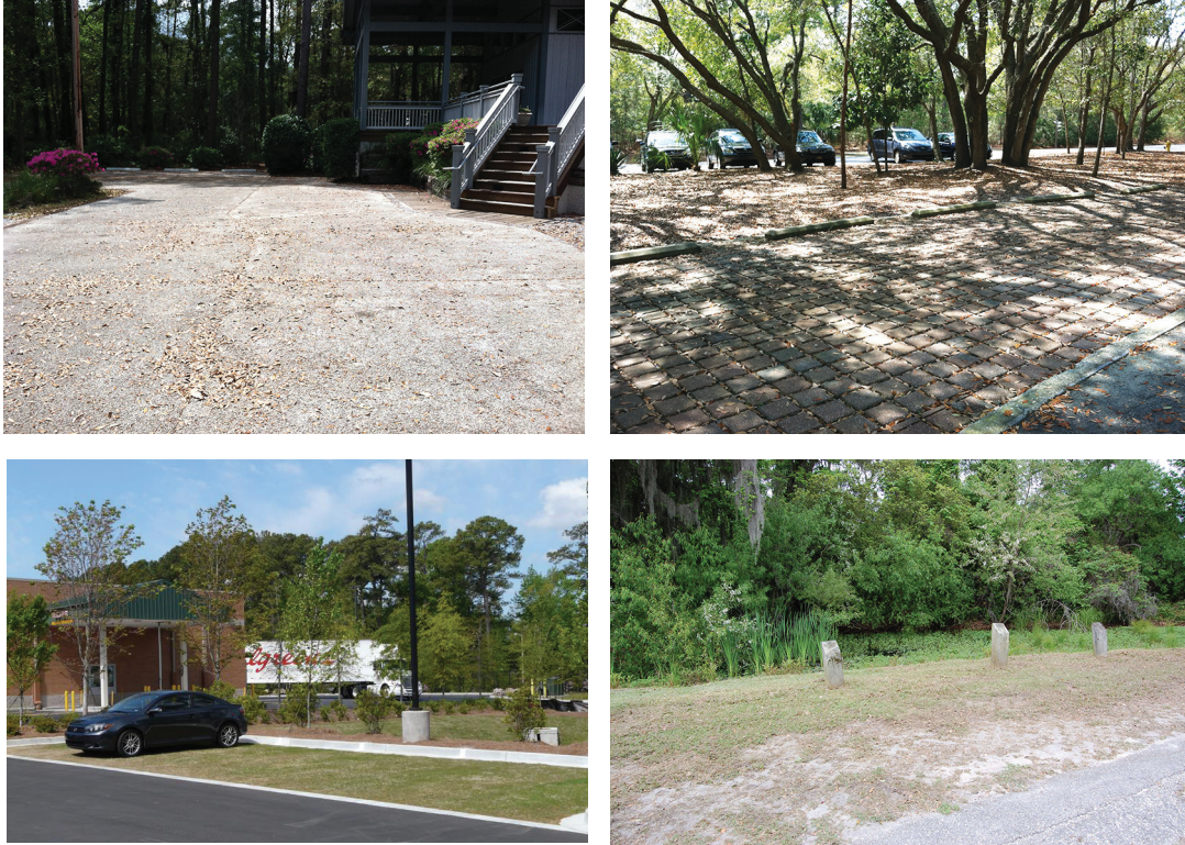
Figure 4.3-3. Various Permeable Pavement Surfaces. Clockwise from top left: (a) Pervious concrete parking lot, Reebok Crossfit Hilton Head Island (Photo: K. Ellis); (b) Permeable pavers at Islanders Beach Park, on Hilton Head Island (Photo: K. Ellis); (c) Concrete grid pavers at Morse Park Landing, Murrells Inlet (Photo: K. Ellis); and (d) Grass pavers at Verizon store in North Myrtle Beach (Photo: Nicole Saladin).
