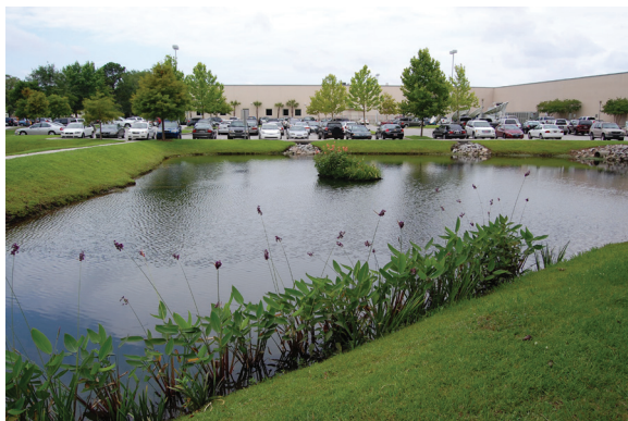
Figure 5.5-2: Native vegetation used in buffer and floating wetland systems in the stormwater pond. (Photo: Kathryn Ellis)
