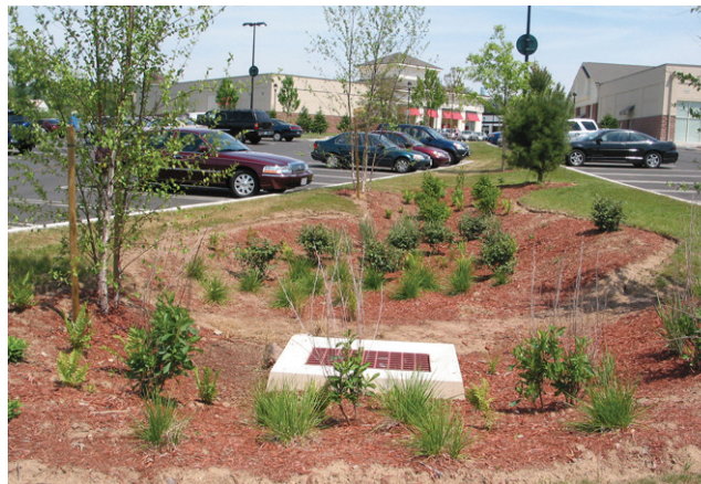
Figure 4.2-1. Bioretention in Parking Lot (Photo: Center for Watershed Protection)
