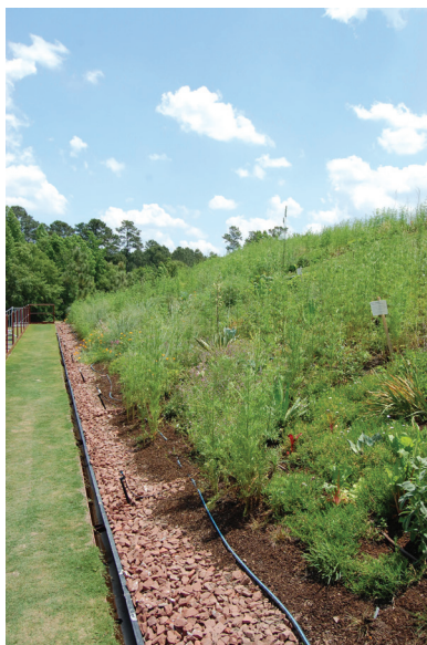
Figure 5.4-2. Walkway, runoff collection gutter, and irrigation system (Photo: Kathryn Ellis)
