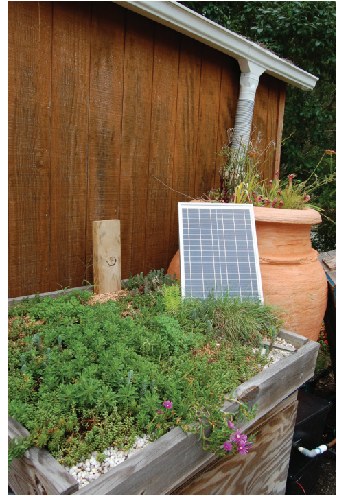
Figure 5.5-3: Demonstration green roof and rain barrel (including a bog garden on top) at the TTC Horticulture building. (Photo: Kathryn Ellis)
