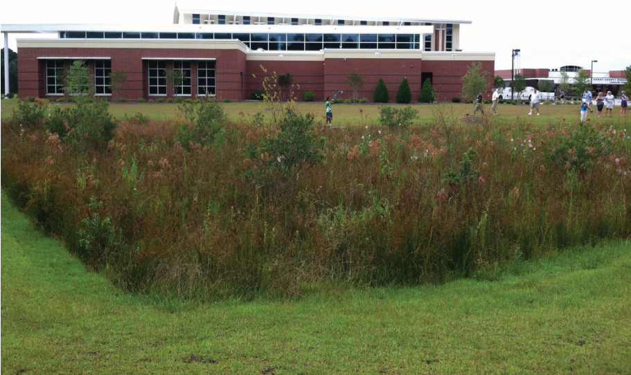
Figure 4.12-1a. Stormwater Wetland at Carolina Forest Recreation Center, Myrtle Beach (Photo: Kathryn Ellis)
