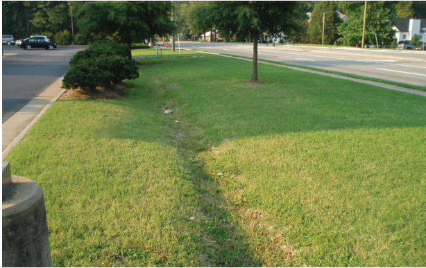
Figure 4.8-1a. Grassed Channel (Photo: CWP)
