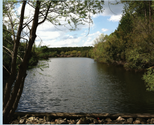
Figure 5.7-1. Stormwater pond at Jarvis Creek Park (Photo: Kathryn Ellis)
