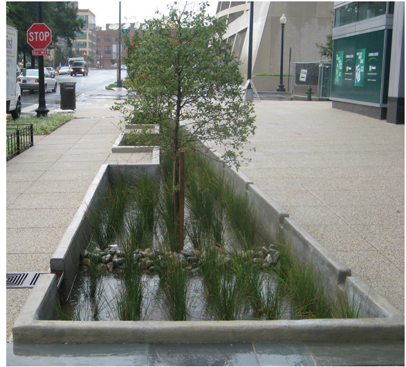
Figure 4.2-7. Bioretention with a Drop Curb (Photo: DC Green Infrastructure http://www.flickr.com/photos/dcgreeninfrastructure/ )
