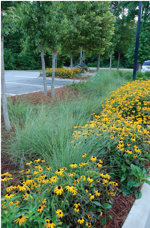
Figure 3.3-9. LID landscaping incorporating stormwater treatment and native vegetation (Photo: Kathryn Ellis)
