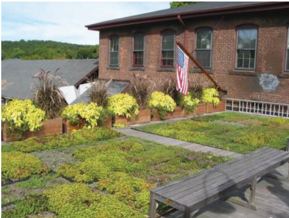
Figure 4.5-1. Green Roof (Photo: Center for Watershed Protection)
