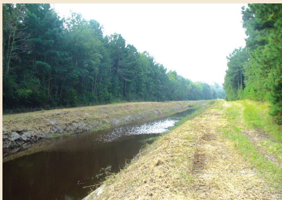
Channel before restoration
