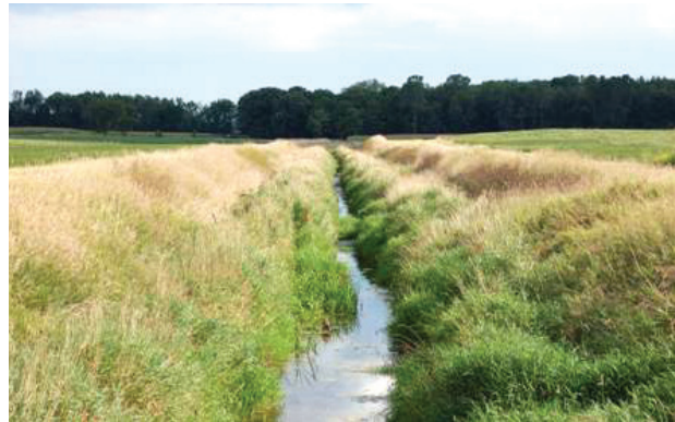
Figure 4.8-1d. Two-Stage Ditch (Photo: Ohio State University Extension)
