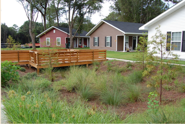
Central bioretention basin serves a dual purpose for community open space and stormwater treatment.
