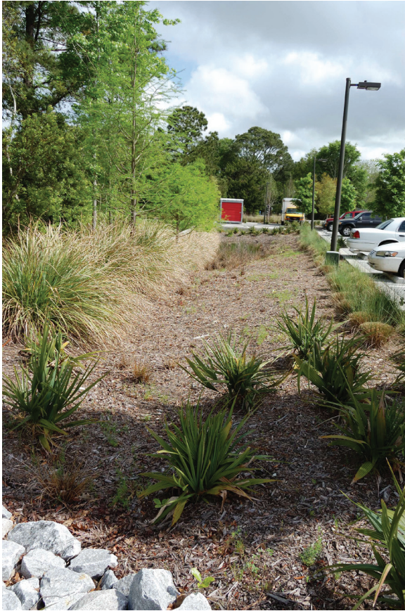
Figure 5.6-3. Bioretention, pervious concrete, and no curb facilitate infiltration of runoff (Photo: Kathryn Ellis).
