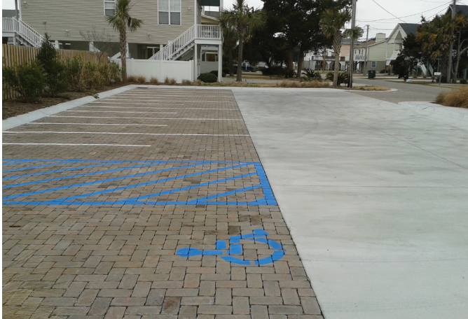
Figure 4.3-1. Permeable pavement parking spaces in North Myrtle Beach, SC (Photo: Travis DuPre)
