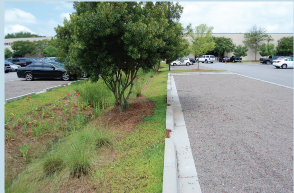
Figure 5.5-1: Pervious parking spaces and bioswale in the TTC Bookstore parking lot. (Photo: Kathryn Ellis)
