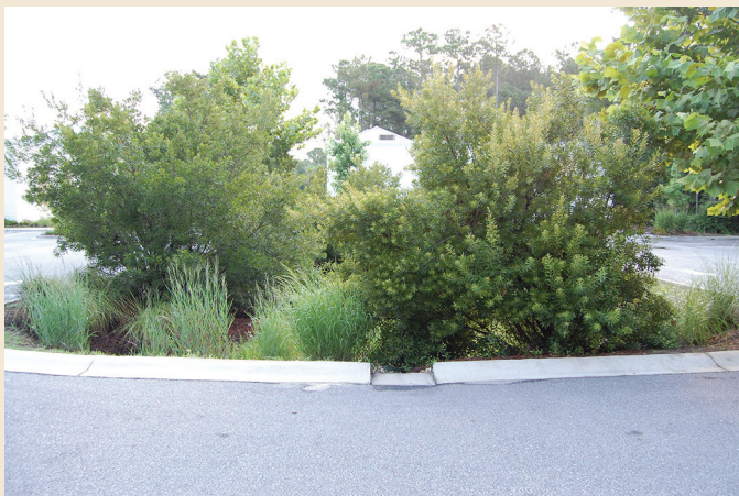
The bioretention cell (left) and swale (right) in grocery store parking lot intercept and treat stormwater runoff.
