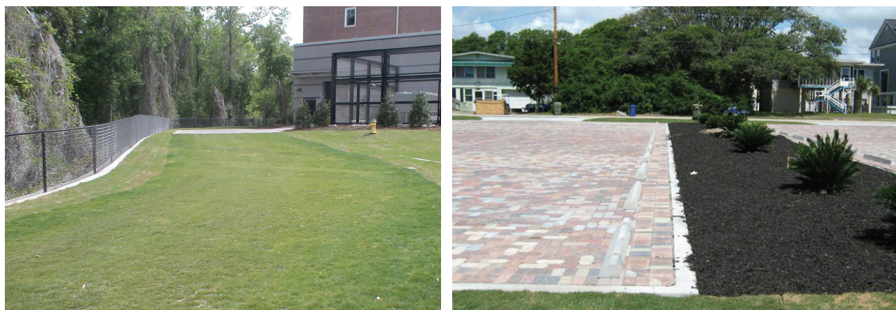
Figure 3.3-5. Local Examples of Alternative Parking Surfaces. Grass paver parking at Coastal Carolina University’s Brooks Stadium (Photo: Karen Fuss, Coastal Carolina University) and pervious pavers installed at the Yaupon parking lot in Surfside Beach (Photo: John Adair, Town of Surfside Beach).
