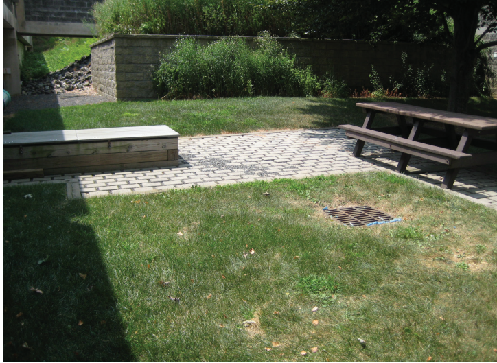
Figure 4.4-10. Example of an Infiltration Trench with Surface Cover (Photo: CWP)
