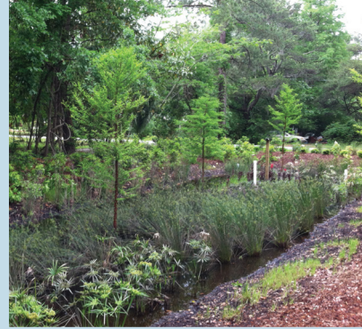
Figure 5.3-1. The larger of two bioretention/wetland cells in Fox Hollow (Photo: Kathryn Ellis)
