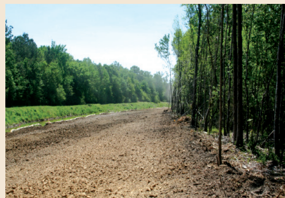
Channel after restoration
