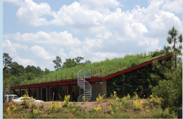
Figure 5.4-1. Green roof on the maintenance building at Moore Farms Botanic Gardens (Photo: Kathryn Ellis)
