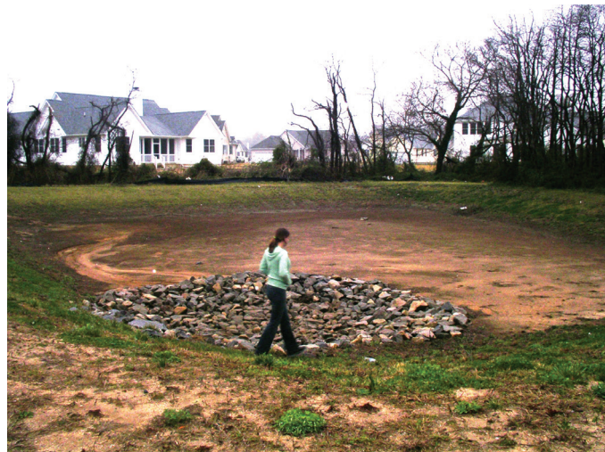
Figure 4.4-4. Infiltration Practices (Photos: CWP). From left to right: (a) infiltration trench and (b) infiltration basin.
