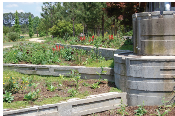
Figure 5.4-4. Cast concrete rain barrel connected to watering troughs for irrigating terraced garden (Photo: Kathryn Ellis)
