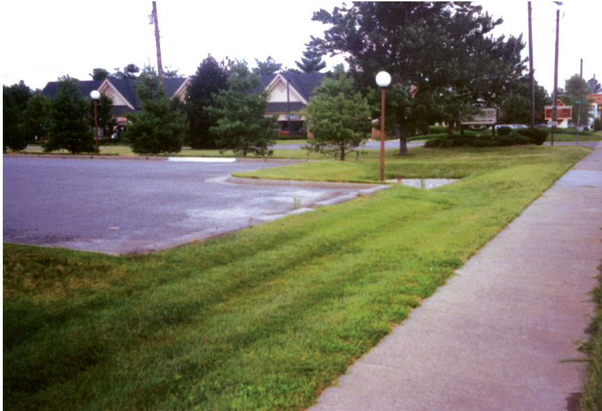
Figure 4.4-7. Infiltration Trench with Grassed Channel Pretreatment (Photo: CWP)
