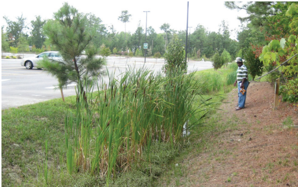
Figure 4.8-1c. Wet Swale (Photo: CWP)
