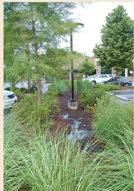
The bioretention cell (left) and swale (right) in grocery store parking lot intercept and treat stormwater runoff.
