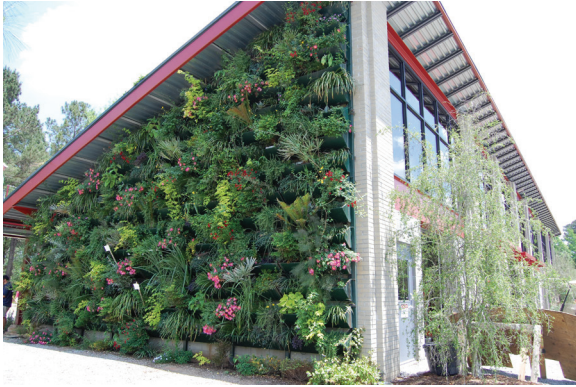
Figure 5.4-3. Other green features include a living wall and south-facing windows. (Photo: Kathryn Ellis)
