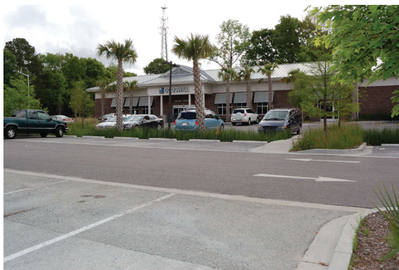
Figure 5.6-2. The parking lot at the Johns Island Goodwill store incorporates bioswales and pervious concrete. (Photo: Kathryn Ellis)
