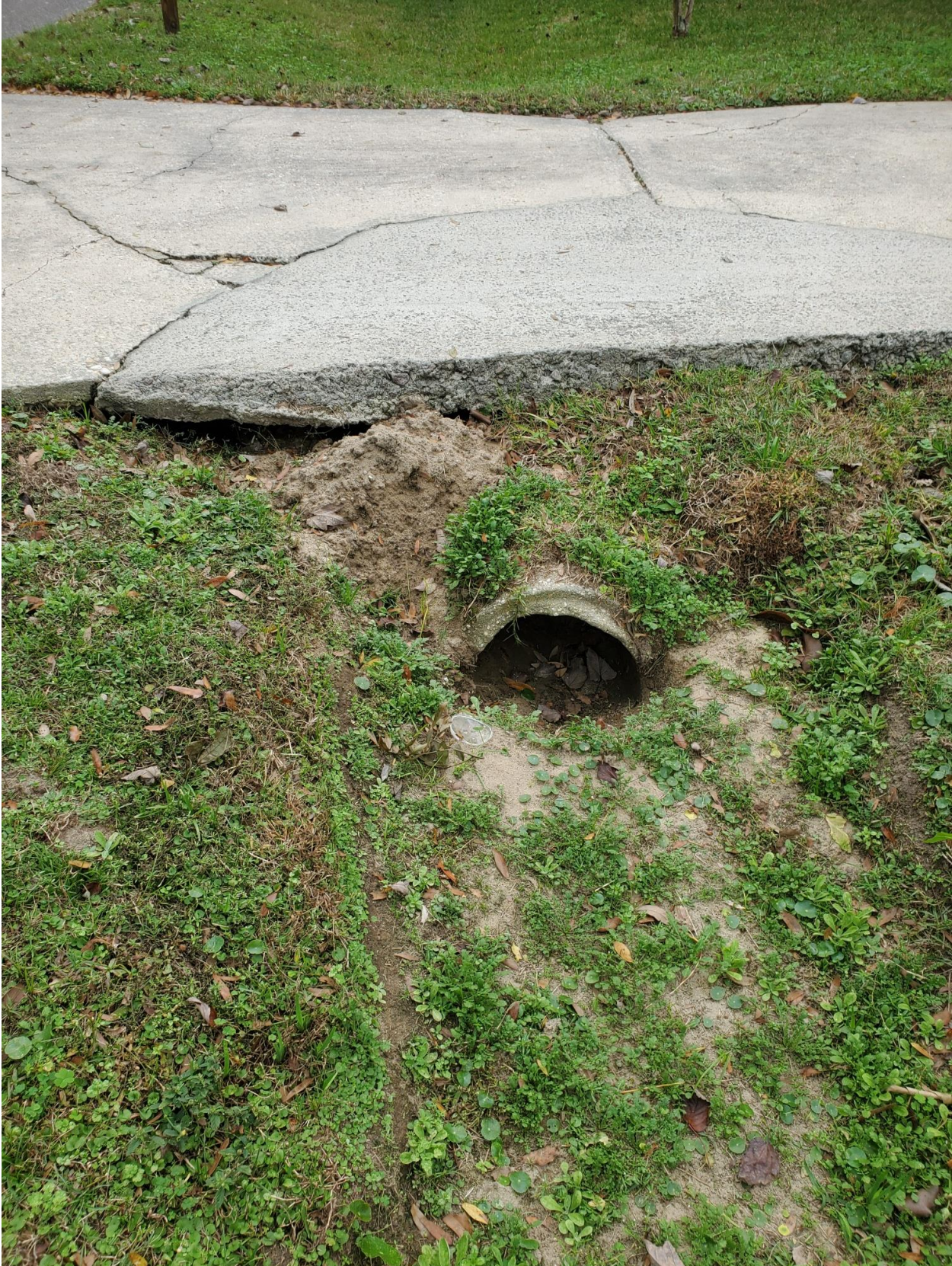
Mt. Vernon Driveway Apron Repair
