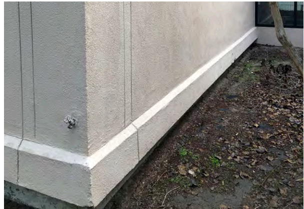
Hose bibs are located on the East elevation
