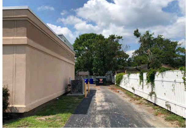
Mechanical units and dumpster access are located north of the building
