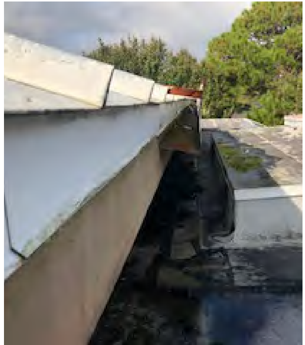
Open ended gutter on the north
