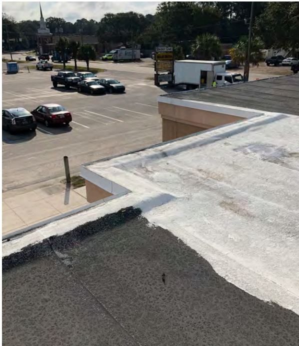
Gravel stop varies in height around the perimeter of the roof
