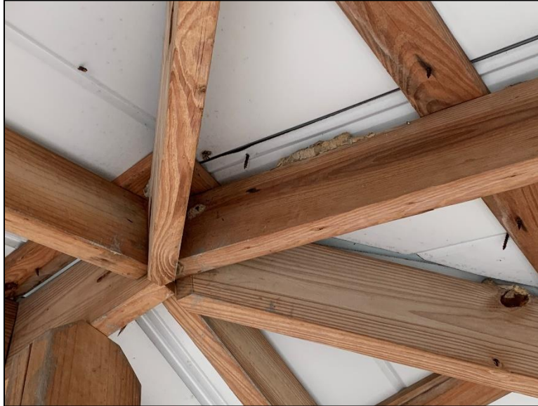
Figure 2.10. Cantilever Rafter Support Other Rafters at Ridge
