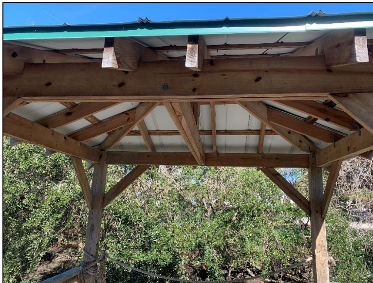
Figure 2.9. Post and Beam Supporting Rafters at Ridge
