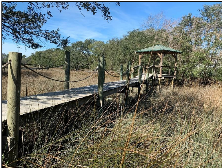
Figure 2.1. Portion of Dock Viewed from the Shoreline
