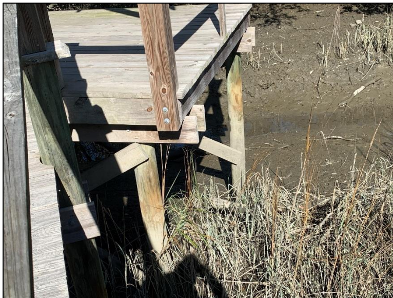
Figure 2.11. Floor Framing for Covered Section of Dock
