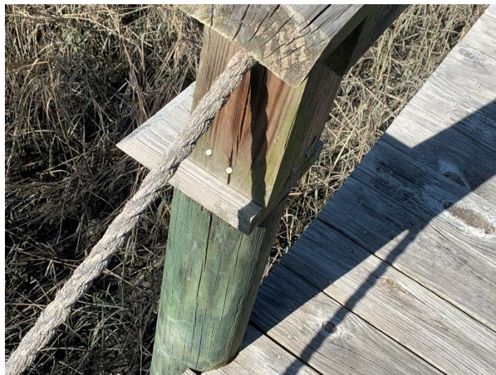
Figure 3.2. Toe-Nailed Railing Post Connections
