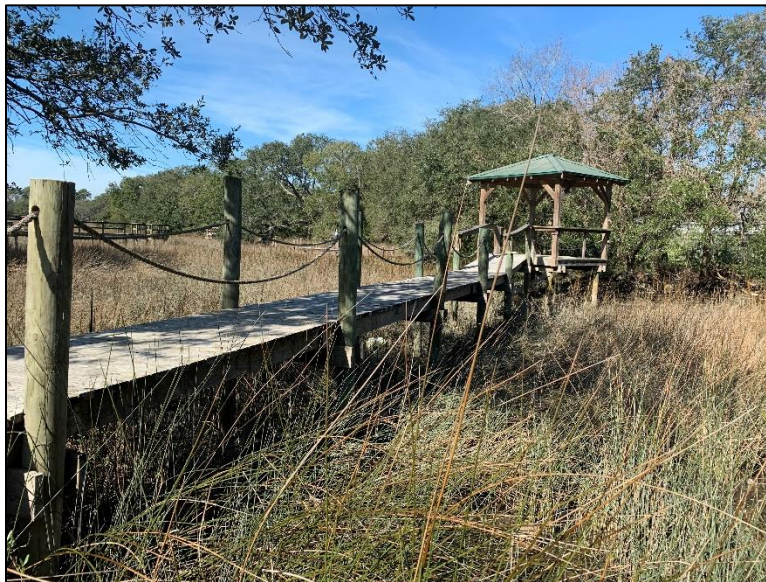
Figure 2.1. Portion of Dock Viewed from the Shoreline
