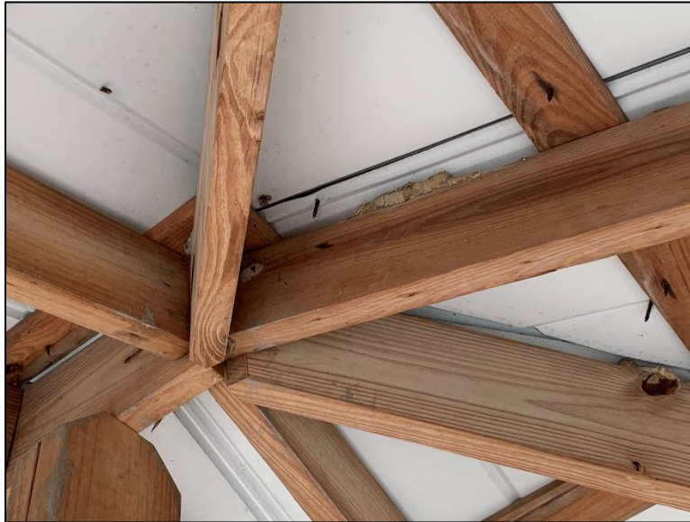
Figure 2.10. Cantilever Rafter Support Other Rafters at Ridge
