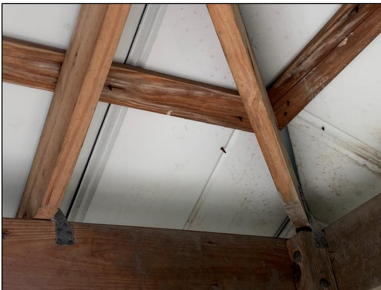
Figure 2.6. Rafters with Hurricane Ties at Ends along the Roof Eave
