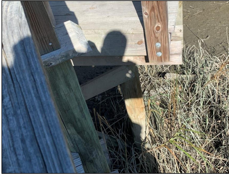
Figure 2.12. Cross-Bracing in One Direction at Bents
