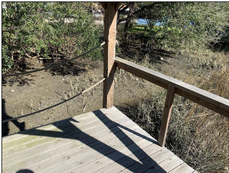
Figure 2.5. Rope Railing on One Side of Covered Section of Dock
