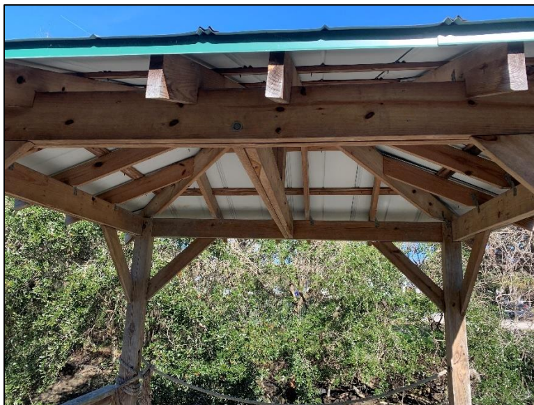
Figure 2.9. Post and Beam Supporting Rafters at Ridge
