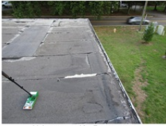
Moisture scan with a Tramex meter.
