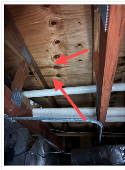
Photo 1 Area by curb with blister may have had minor signs of moisture damage.
