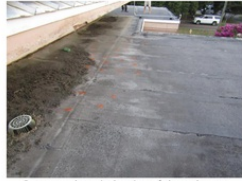
Dots sprayed at point locations of elevated meter readings.
